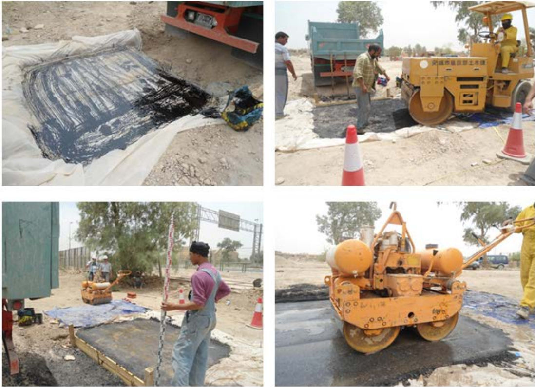
Figure (4) Asphalt pavement works (Flexible Pavement).
