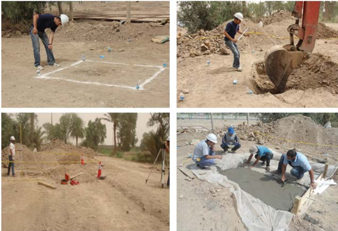
Figure (3) Excavation and casting concrete works (Rigid Pavement).
