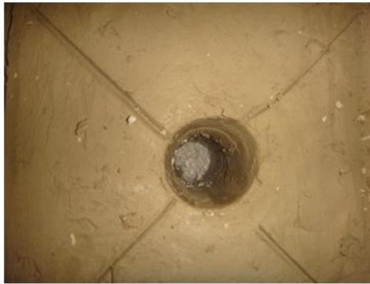
c): Pouring of crush stone
