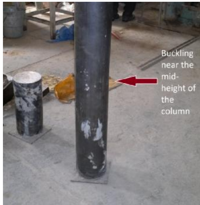
Figure. 10 Failure of the long column
