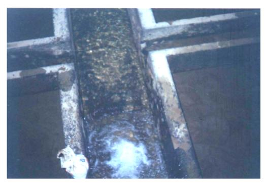
Plate 2: Sand in the Wash Water Trough is an Indication of the Escape of this Material Due to Excessive Air Scour.
