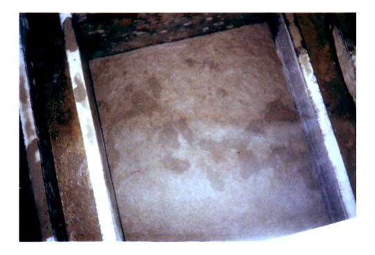
Plate 1: Mounds and Holes in the Filter Bed Suggest Probability of Problems in the Gravel and Under Drains.
