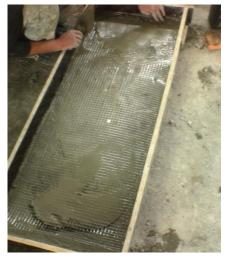
Fig 2: Placing the wiremesh
