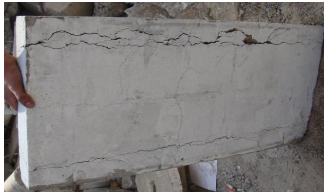
Plate 5. Bottom failure surface of CC slab without fibres.
