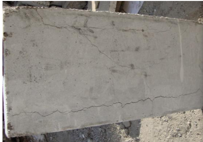
Plate 7. Bottom failure surface of CC slab with 0.14% fibres.
