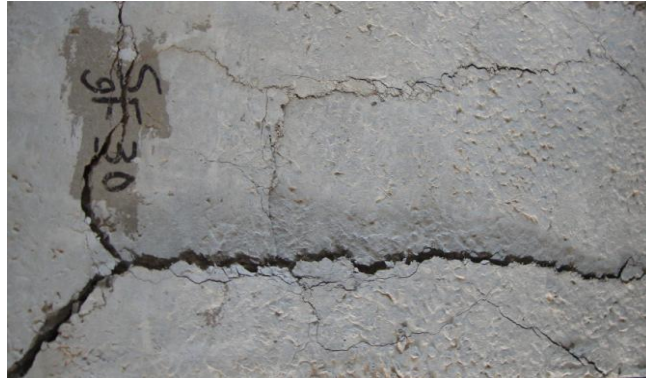
Plate 3. Top failure surface of SCC slab with 0.07% fibres.
