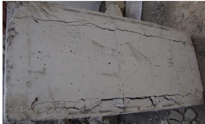
Plate 4. Bottom failure surface of SCC slab with 0.14% fibres.
