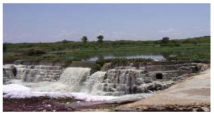
Figure (2) Hyderabad, India–95 percent of the waste water is disposed untreated in the Musi River, wastewater being diverted over weir into irrigation canals.
