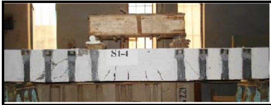
Figure 9: Crack pattern at ultimate failure of specimen S1-4
