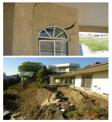
Fig. (1): Structural failure for light weight buildings constructed on collapsible gypseous soil.
