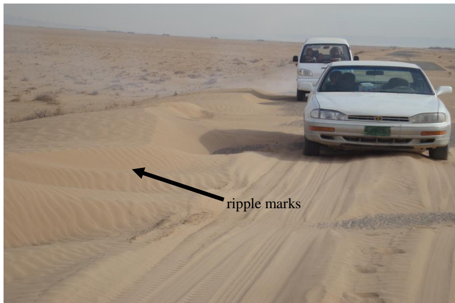
Fig.6: Shows Recent ripple marks sedimentary structure in sand dunes which cover the paved roads.
