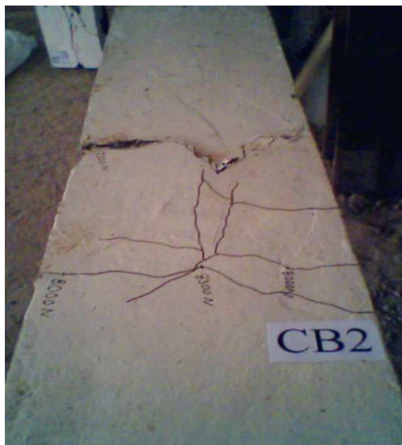
Figure (6): Cracking of concrete at Beam CB2
