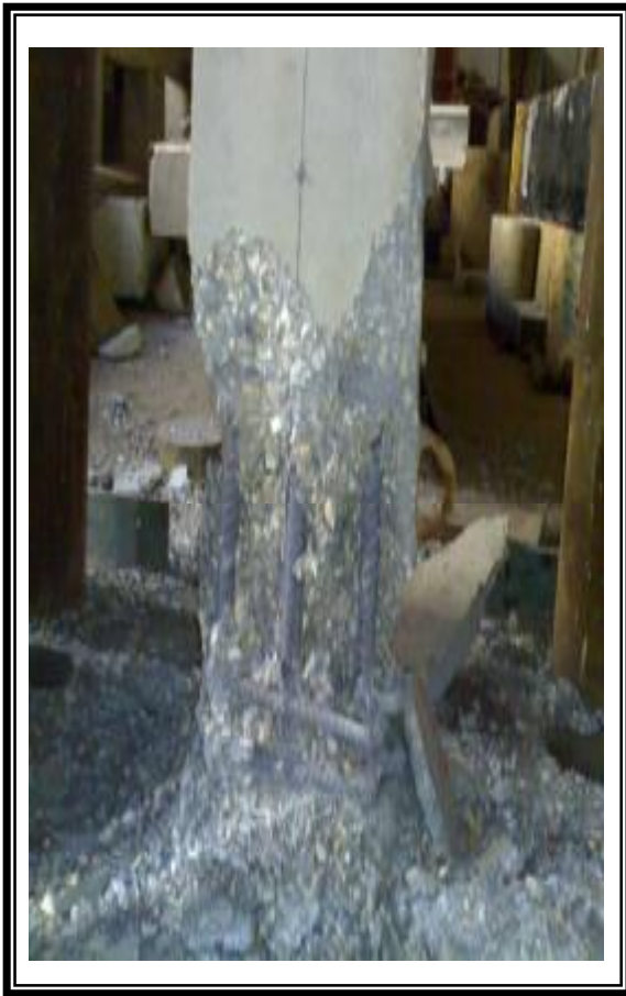
Figure (9) Failure Mode of Column A 3 B 1 C 1
