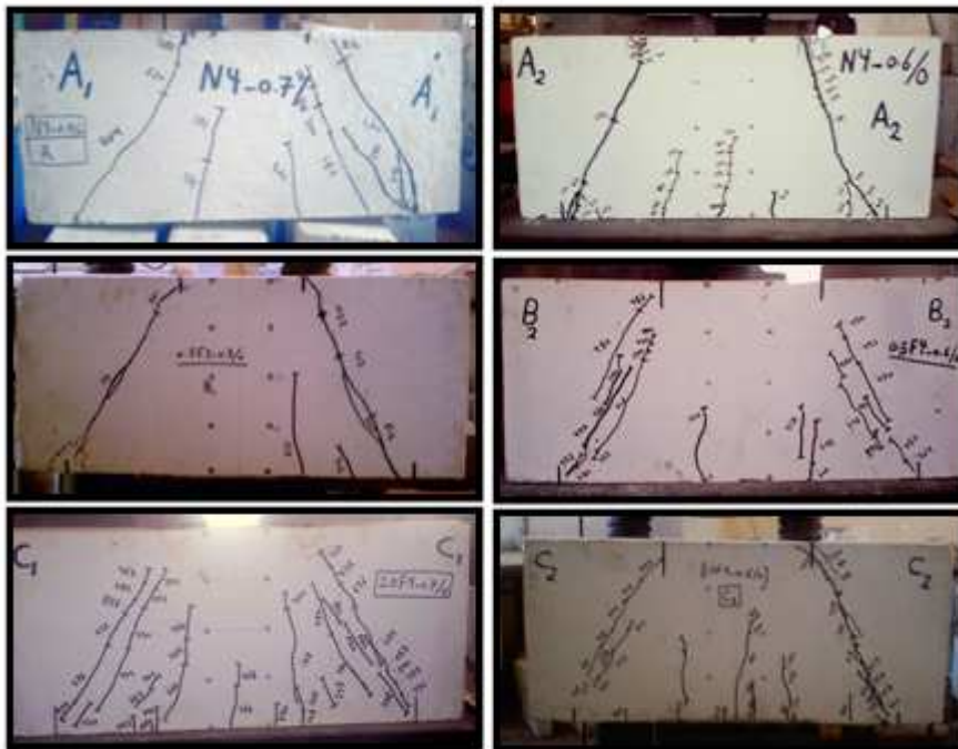
Figure (11) Crack patterns at failure of deep beams without web opening
