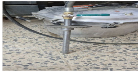
Plate 4: The tube for cement grouting
