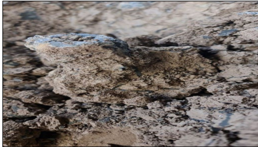
Plate 9: The heated treated soil with cement grouting content 0.5 of water cement ratio
