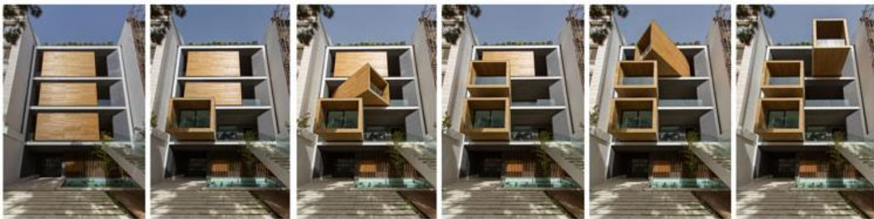
Figure (11): Shows the transformation in The Tehran house that turns with the seasons, Source: (Archdaily, 2014).
