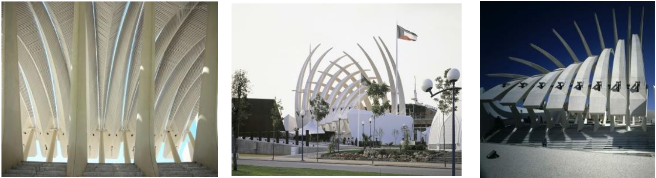
Figure (10): Shows a retractable roof for the Kuwait Pavilion, Source: (Asefi, 2012).
