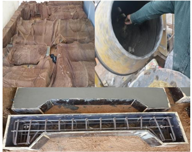
Figure 2: Preparation of moulds, mixing and curing operations
