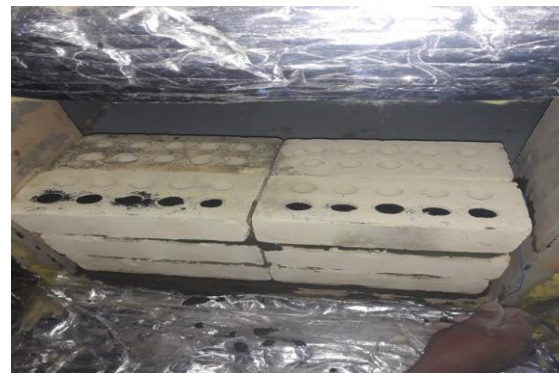
Figure 9. Put the tire scrap power in the line of the outer holes during construction
