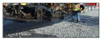
Figure 3. Porous asphalt paving[45]
