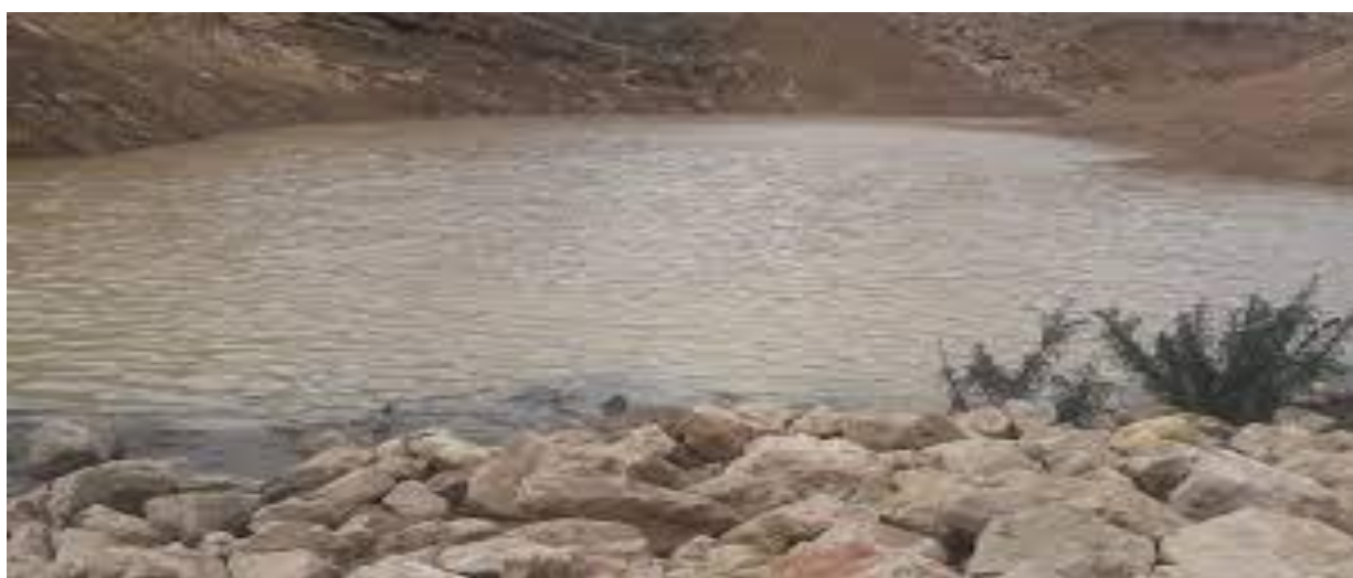
Figure 10: Constructing stone dams to hold and harvest water within arid regions
