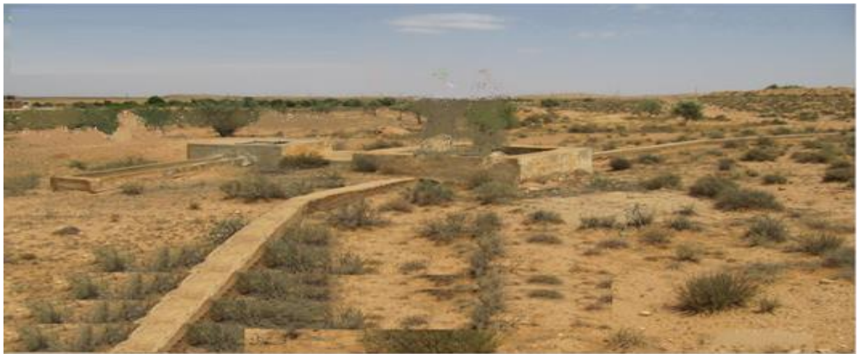
Figure 13: Technologies for holding water towards ground tanks to harvest rainwater in dry areas
