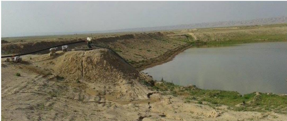
Figure 12: Conserving water within the site to harvest rainwater and prevent surface runoff within arid areas
