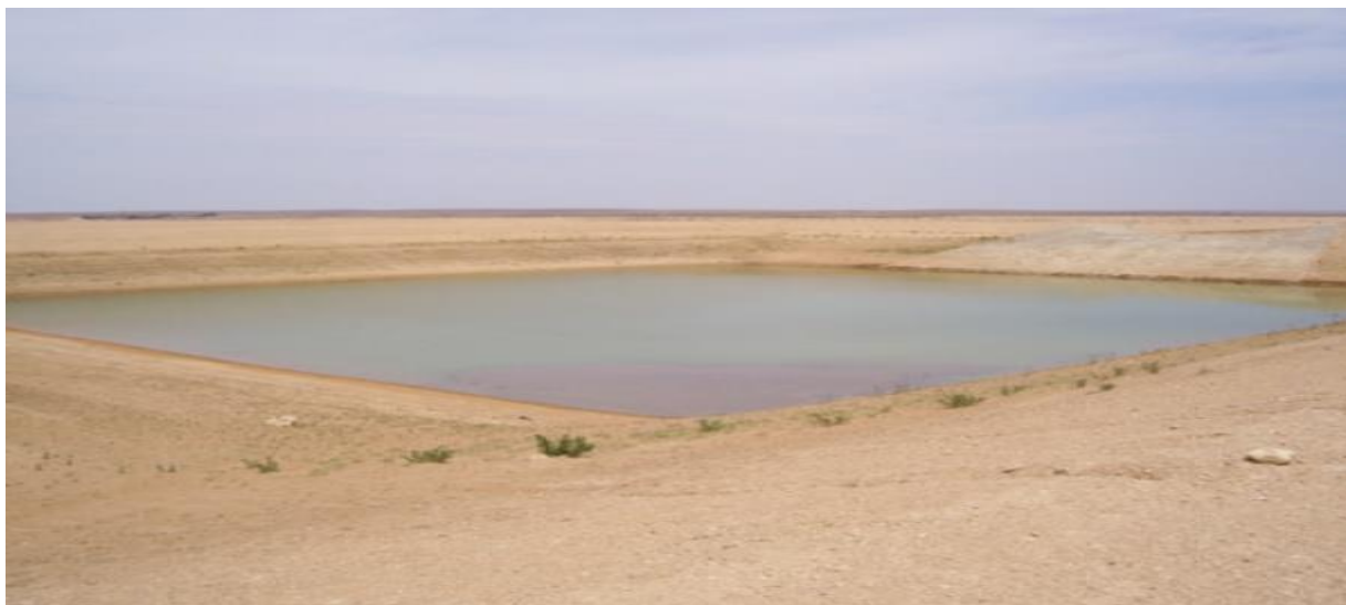
Figure 9: Construction of pits to harvest water within the flat areas
