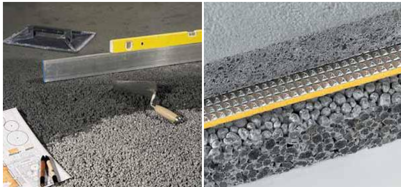
Fig.3 Lightweight Concrete( Laterlite technical Assistance, 2006)
