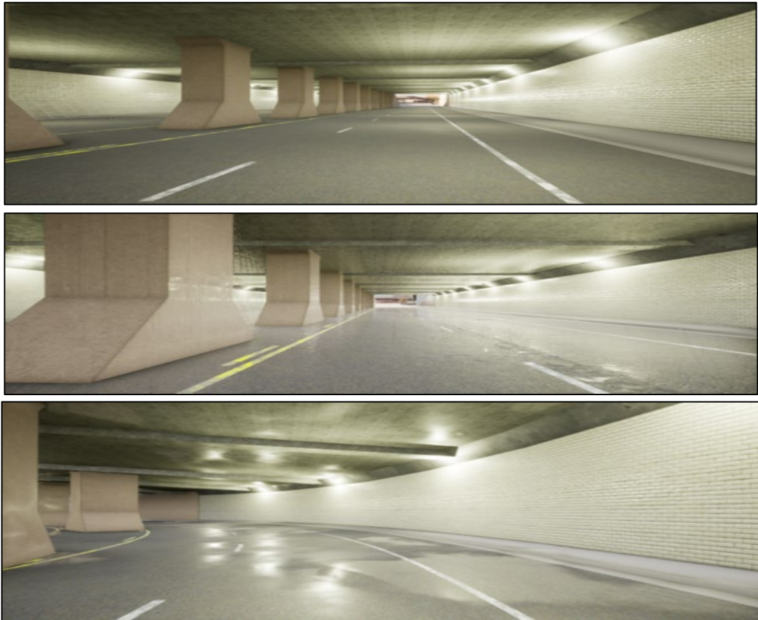
Figure 7: RGB image of the Tunnel in bright sunny, hard rain noon, and wet cloudy noon, respectively [24]
