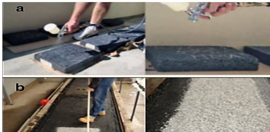
Figure 4: (a) The TiO 2 solution spraying process (b) the painting process of TiO 2 solution [43]
