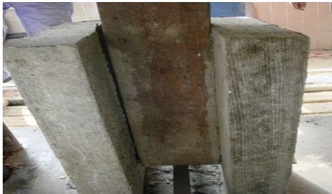
Figure 5: Failure of push-out specimens by the separation between timber and concrete
