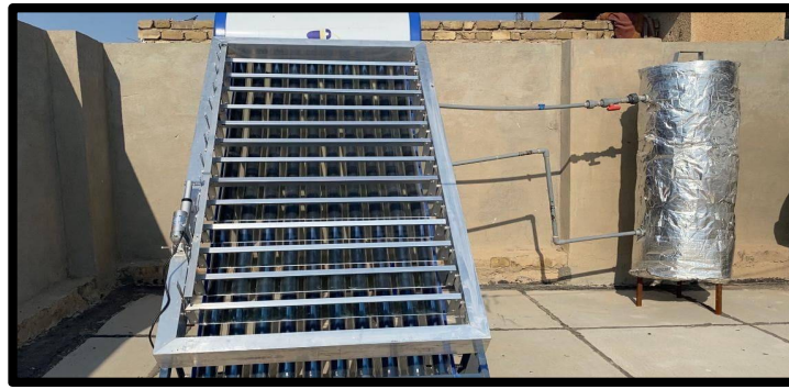
Figure 1: Evacuated tube solar collector
