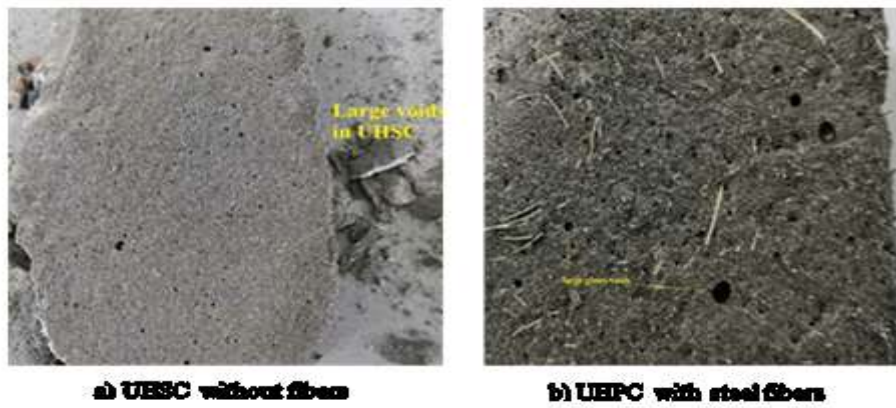
Figure 5: The voids in UHSC and UHPC because of autogenously shrinkage UHSC: Ultra-high strength concrete
