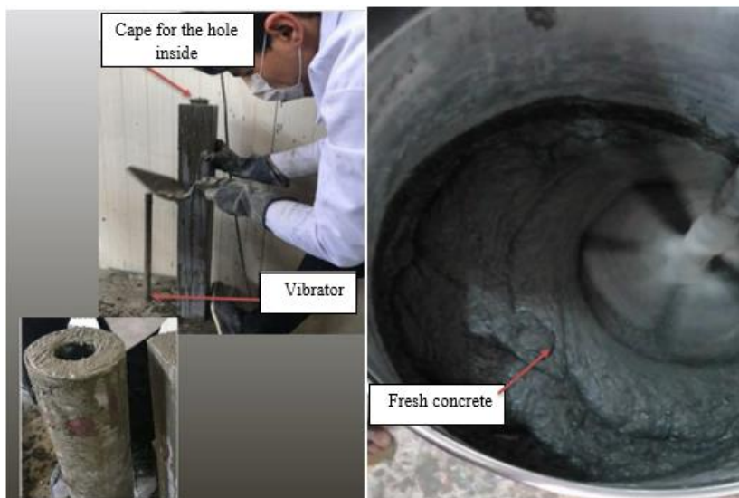
Plate (3) Mixing, placing and compacting of concrete.
