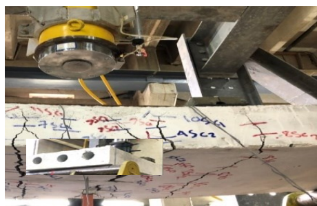
Figure 7: Bottom face of tested slab 3V75NR2 under repeated load pattern (R2)
