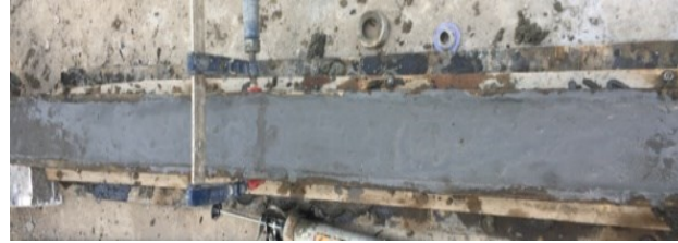
e. Finally, the beams
