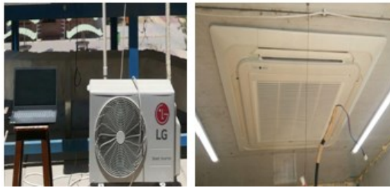
Figure 6: Inverter 4-way cassette air conditioner
