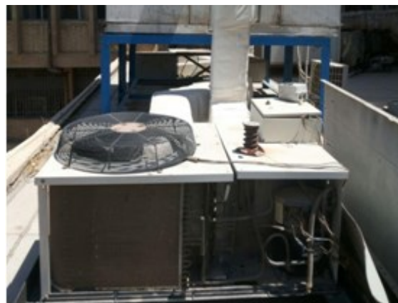
Figure 13: Packaged unit
