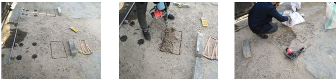
Marking and excavation process
