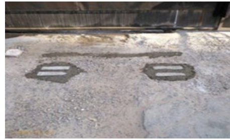
Fixing process of sensors into the holes Figure 5: Continued
