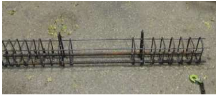
Figure 2: Steel reinforcement details
