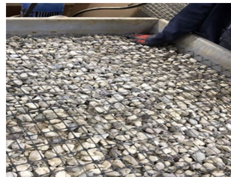
Figure 6: Base reinforced with geogrid
