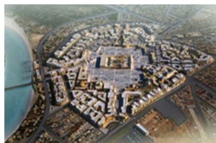
Figure (2) the winner project of Kadhimiyadevelopment by the Diwan Bureau for Architecture [11]
