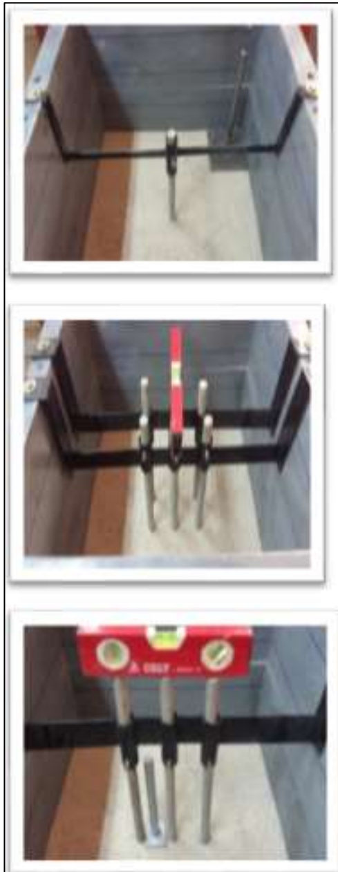
Plate 4: Fixed piles by steel plates
