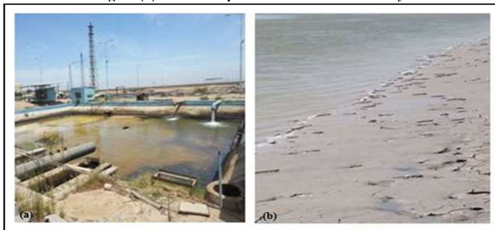
Figure (3) Collection basin unit and wastewater treatment in the Shuaiba refinery before thrown into Shatt Al-Basra River; (b) Polluted area in Shatt Al-Basra and nearby banks
