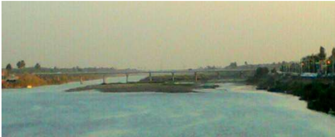
Figure (2): Al- Hindiya second bridge
