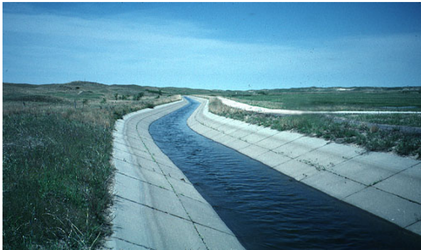
Figure(2): Concrete lining for irrigation canal.
