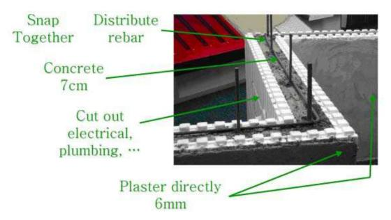
Figure (2)the main structural wall elements
