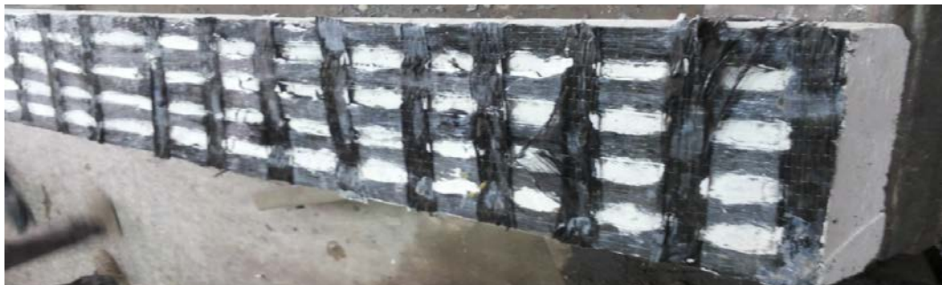
Figure (8.4) Cracks pattern after failure for slab SHS3
