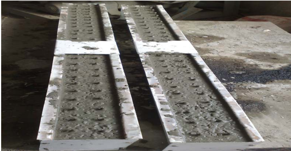
Plate (3)Bonded Beam Casting
