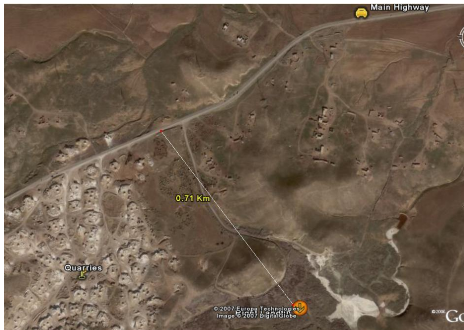
Figure (4). Relationship of the west landfill site to its surroundings
