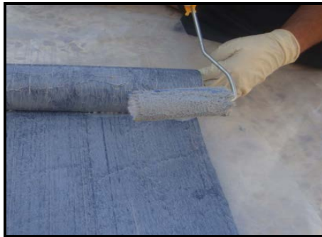
Plate (2) Specimens retrofitting process
